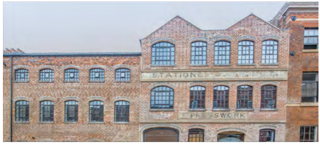
Above, Clement W20 bespoke steel windows at Comet Works, Birmingham.
